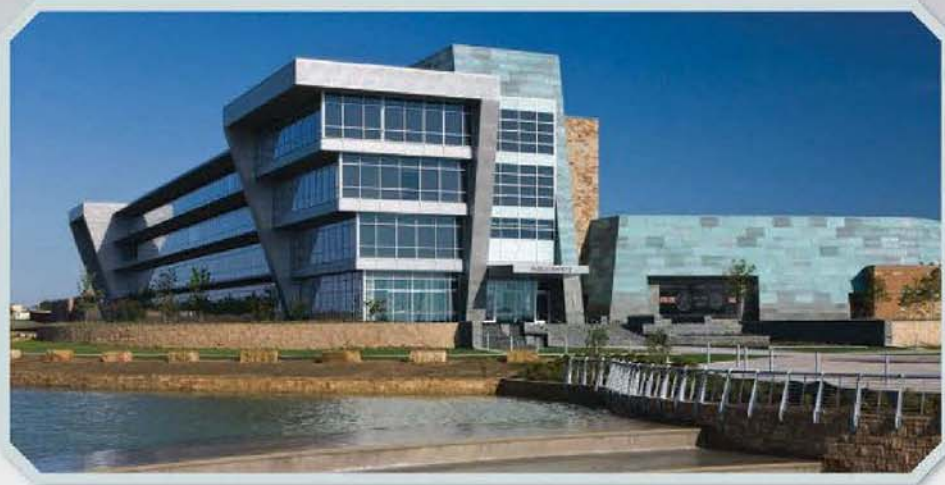
■ Grand Prairie, Texas Public Safety Facility
